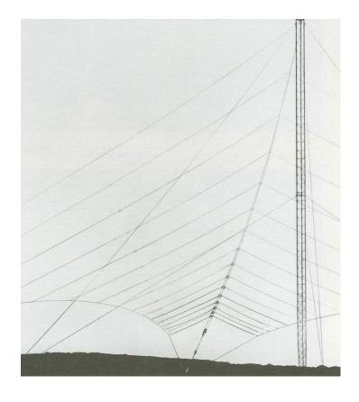
Power ratings of up to 20 kW average, 40kW peak are available. A single balun transformer converts the 200 ohm antenna feedline to a 50 ohm coaxial input.
